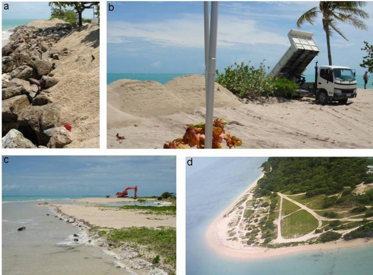
Figure 7.2: Warraber sand relocation, receiving area (a,b), extraction area (c,d).
