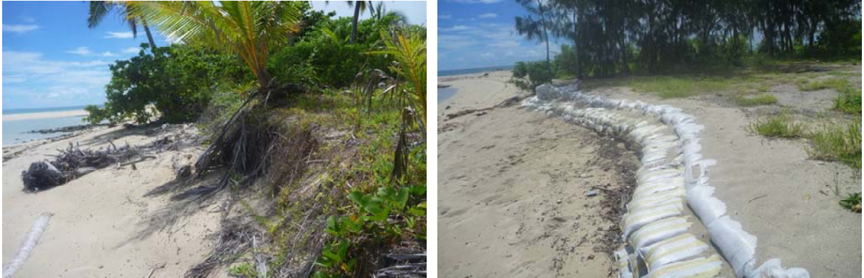
Figure 7.4: Erosion of the south-western corner of Poruma, showing sandbags placed by the community.
