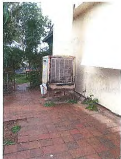
Figure 11 Evaporative Cooler requires replacement
