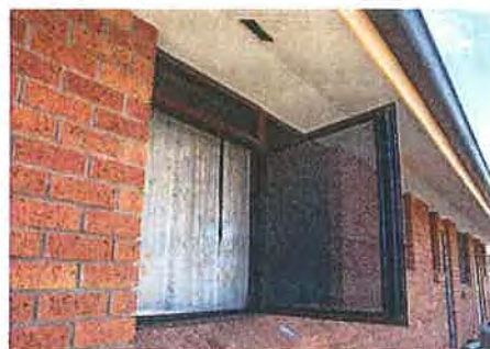
Figure 5 CrimSafe Security Screen damaging eaves of property
