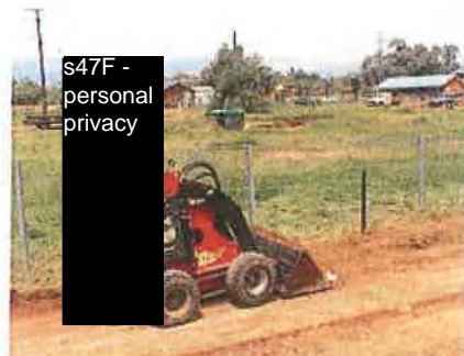
Figure 14 - Grading Driveway
