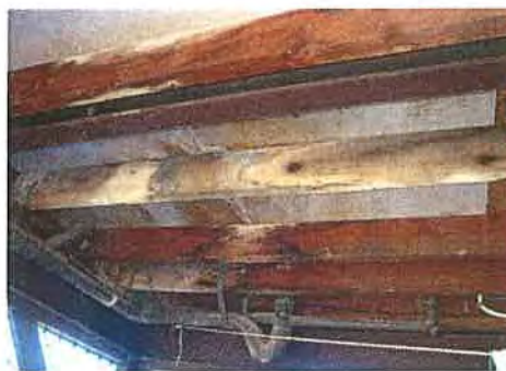
Figure 4 Water Damage
